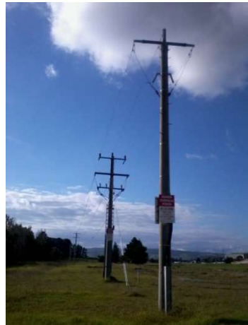
Pole 1&2: looking North
