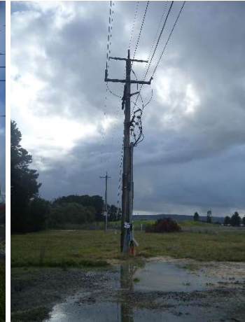
Pole 4&5: Looking North
