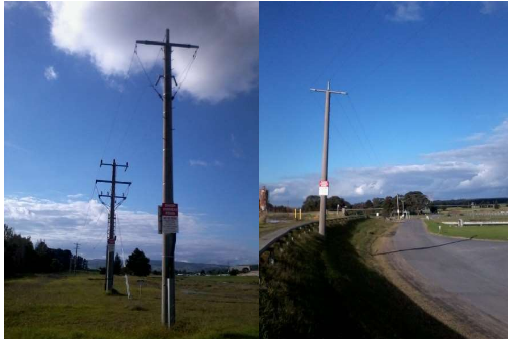
Pole 1: looking North
