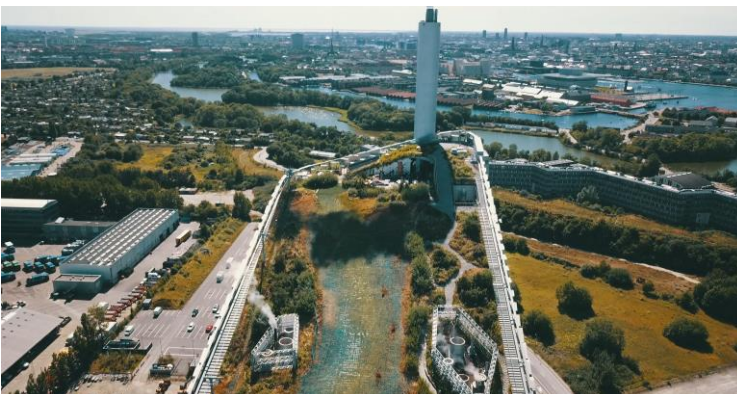
CopenHill EfW facility in Copenhagen with technology installed by Babcock & Wilcox
