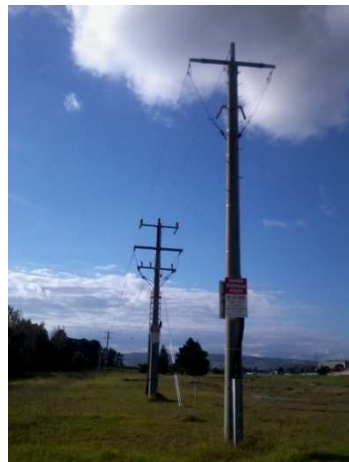
Pole 1&2: looking North
