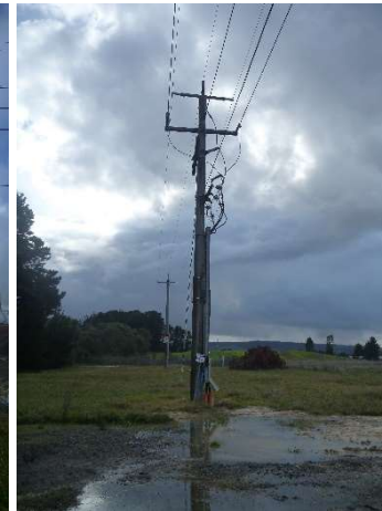
Pole 4&5: Looking North
