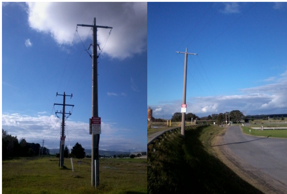
Pole 1: looking North
