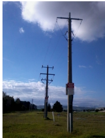
Pole 1&2: looking North
