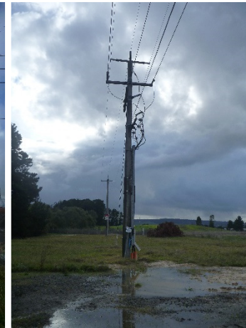
Pole 4&5: Looking North
