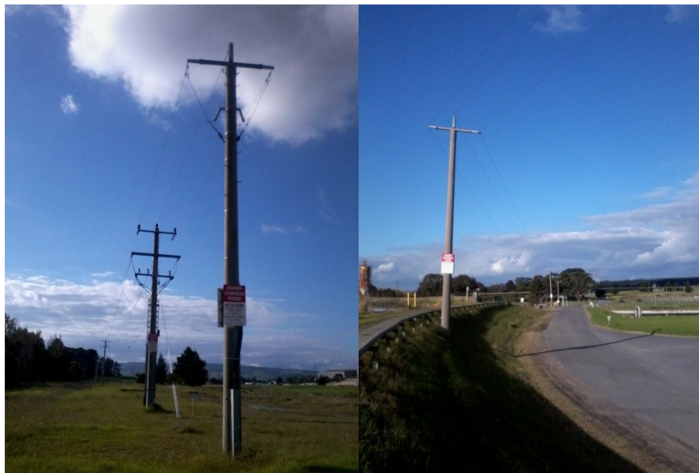
Pole 1: looking North
